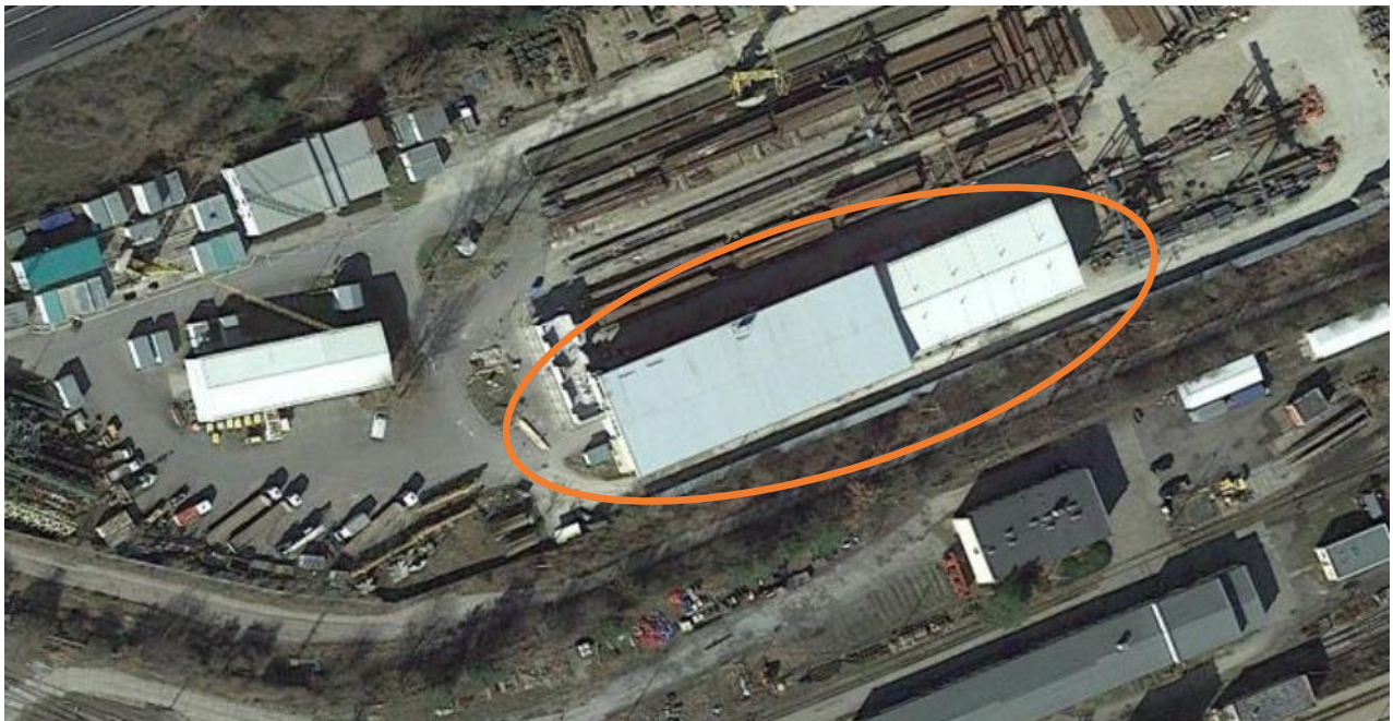
Figures 3 - Ground production hall from bird's eye view
