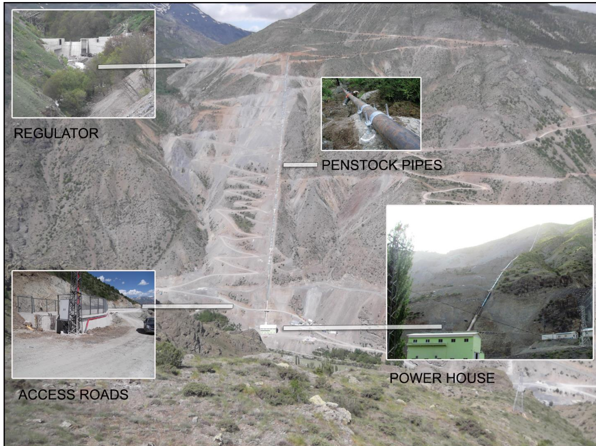
Figure 1. Hydropower (HPP) applications rehabilitation project (Ispir-Coruh basin)
