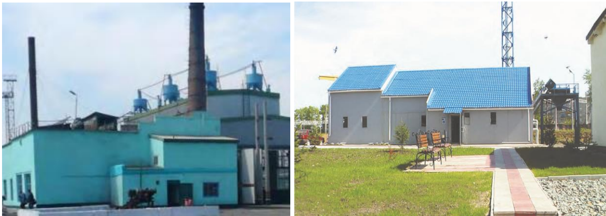
Figure 5. Old boiler-house (left picture) and CHSU-3.0 (right picture)
